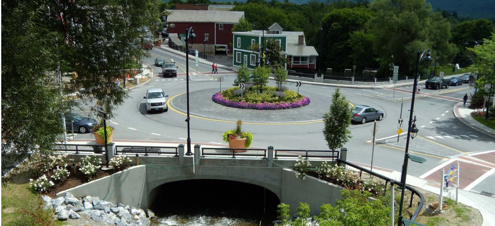
Manchester Roundabout, Manchester, Vermont
