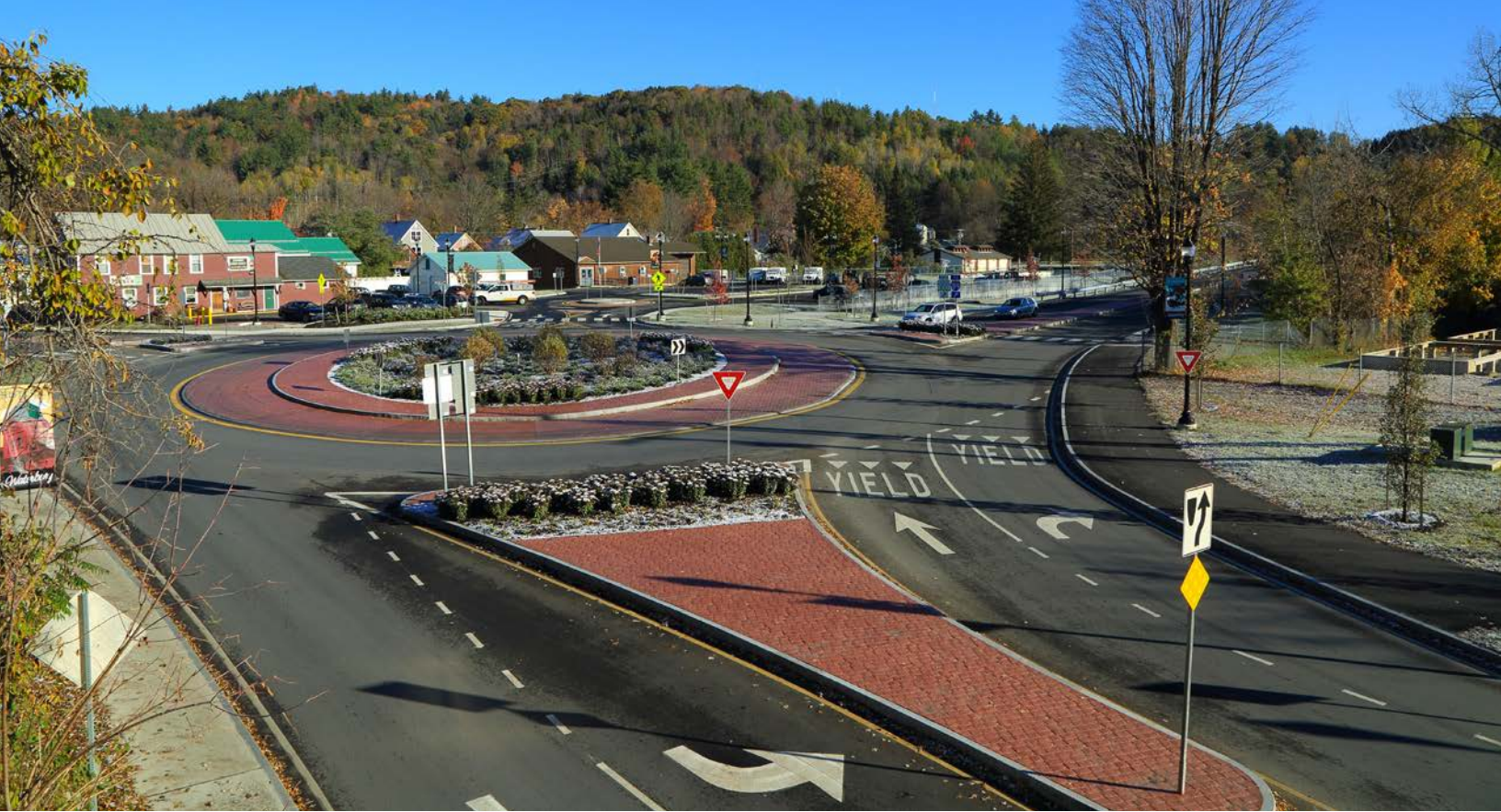
US2/VT 100 Intersection Improvements, Waterbury, Vermont
